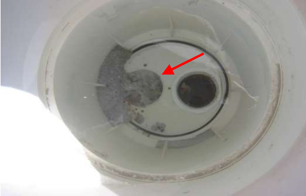
Concrete in pool skimmer.
