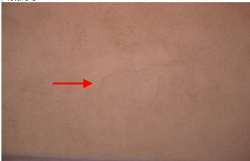
Work on stucco patch on East wall outside master bathroom.
